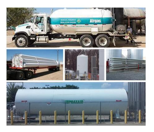
This first image shows you the various ways you might get raw materials for your atmosphere furnaces. On the top, you'll see a picture of a delivery vehicle and storage tank for anhydrous ammonia (NH<sub>3</sub>). NH<sub>3</sub> is ammonia intended not to contain water, to break down into a dry atmosphere. In the thermal processing industry, buyers of NH<sub>3</sub> would buy metallurgical grade NH<sub>3</sub>, which is the highest quality, intended to break down cleanly in a dissociator.
